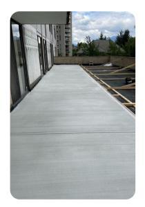
The only project that is still ongoing is our renovation work on the third floor. We have removed the existing pavers and added two new membranes on top of the existing layer to improve waterproofing; we have then poured concrete above them instead of adding new pavers in order to create a safer environment with less tripping hazards. While the heavy duty work is completed, we are now working on the final touches, such as procuring new planters and pots that can be
